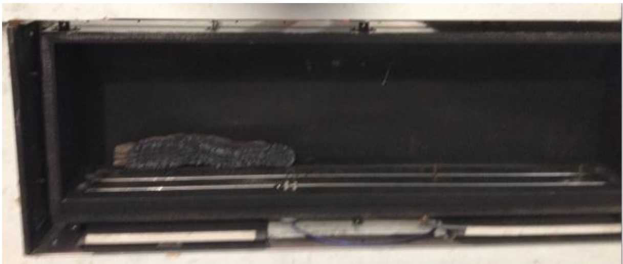
Rear left log in position
